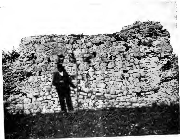
4. A PIECE OF THE MURO PERTUSO BETWEEN TWO BUTTRESSES View from the south
